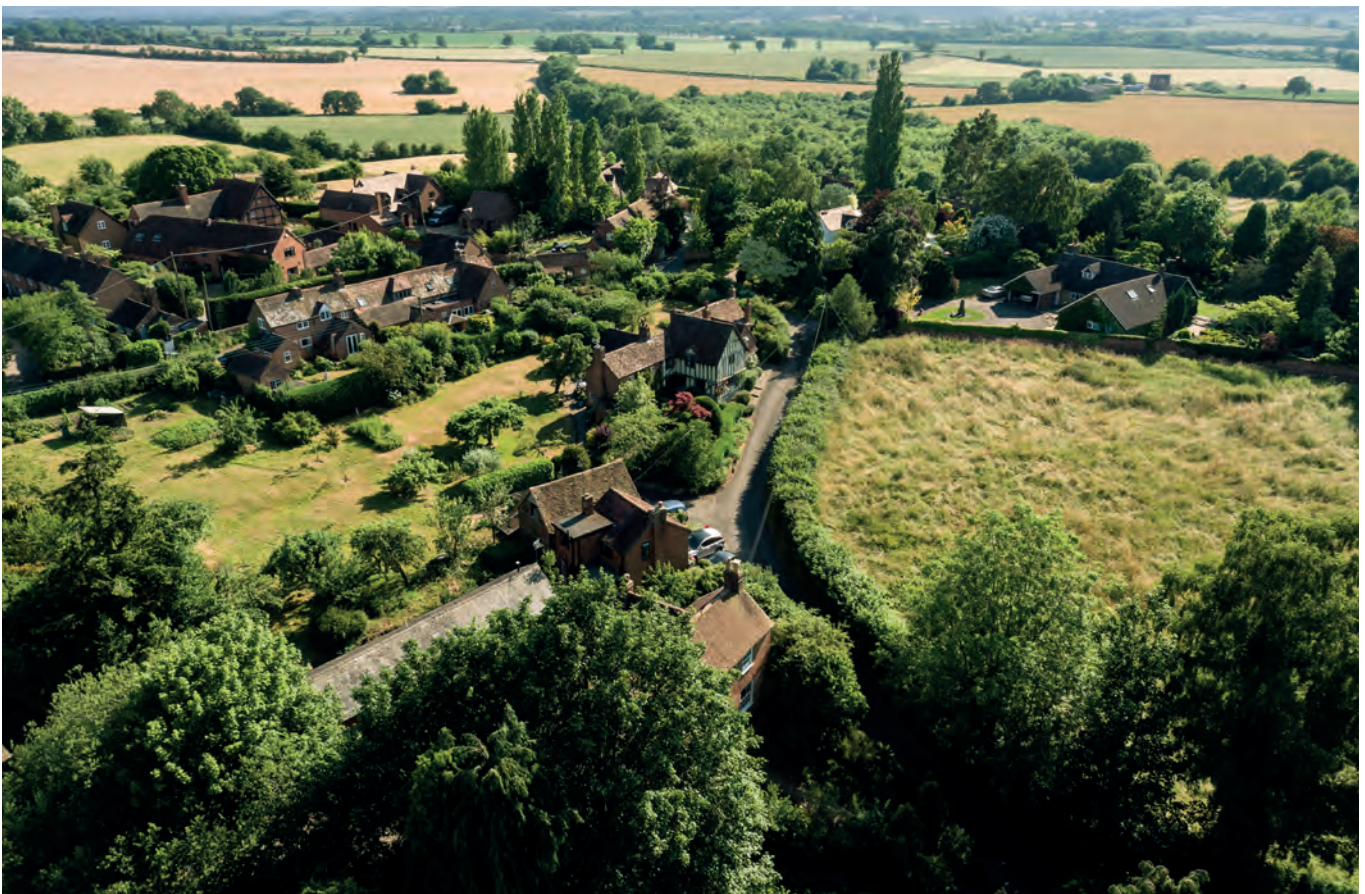
Church Lane heritage properties, looking south from church
